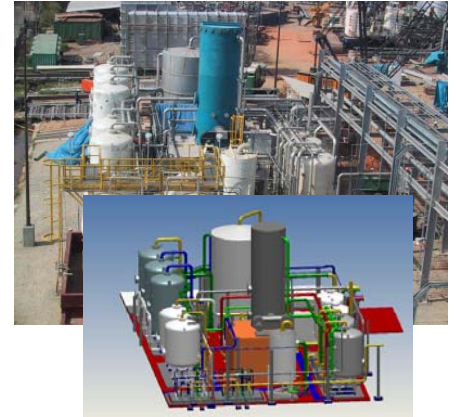
A water pretreatment plant with desalination in Trinidad, and its MPDS model
