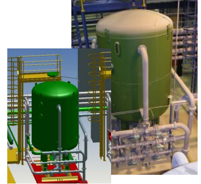
An activated carbon filter unit at the Elbistan power plant in Turkey, and its 3D model in MPDS
