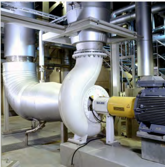
Circulation pump AHLSTAR™ APP pumping black liquor in the evaporation plant of a chemical pulp mill
