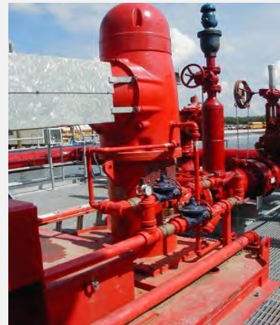
The JF vertical fire pump is ready for instant operation, taking water from wells, reservoirs or other reliable sources.
